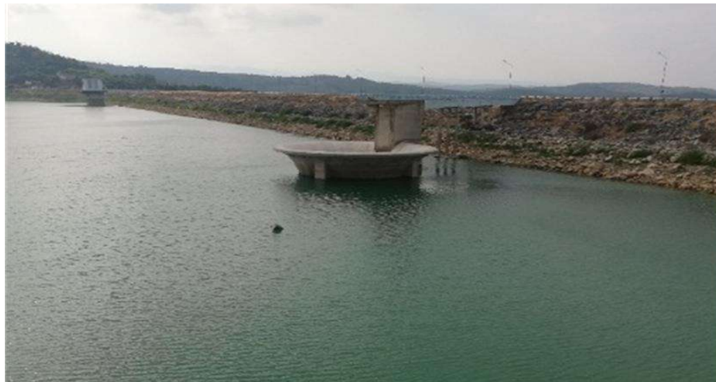
Figure 3. 16 Tishreen Dam Lake (clear sight).
